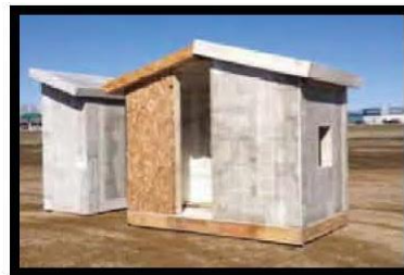
½ of the building using OSB + Closed Cell Polyurethane + OSB SIP and ½ of the building (plus outer building) using TGS SIP
