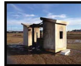
Only the TGS SIP buildings survived.
